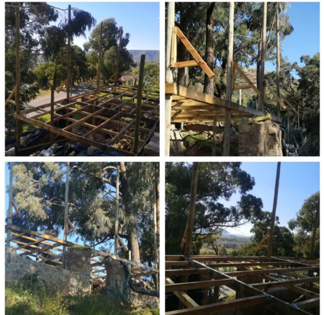
Progress made in building two classrooms.
