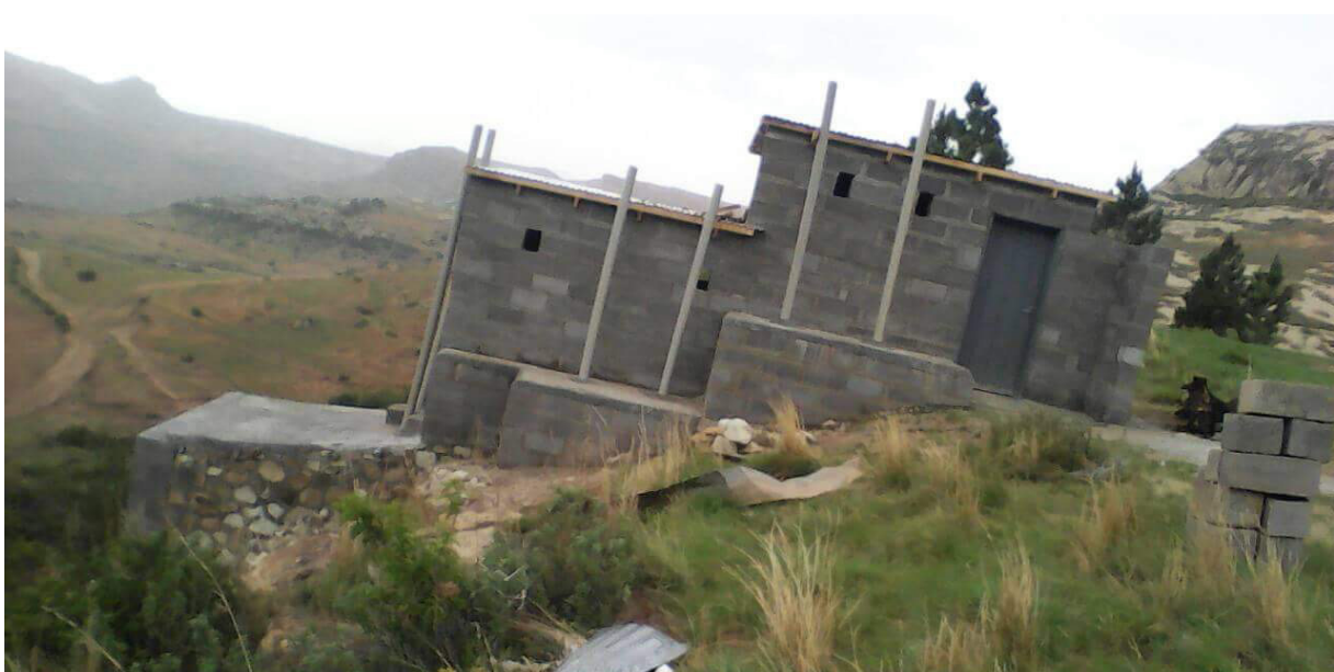
The new latrine structure in Ketane
